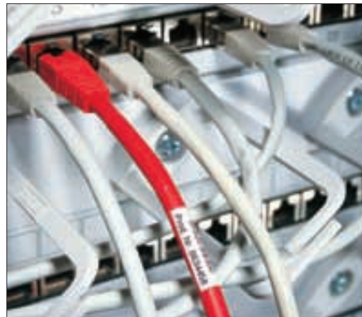
Self-laminating labels offer an excellent protection against abrasion and environmental impact.
