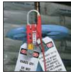
Lockout gate valves
