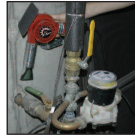
Thaw Frozen Pipes
