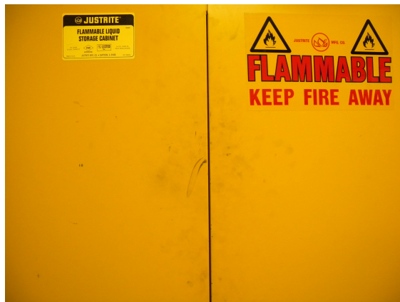
Figure 1-13. Flammables should be stored in an appropriate cabinet to help prevent unintended fire.
