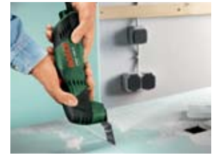
Trimming plasterboard.
