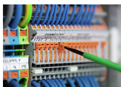
Pivoting a knife disconnect.
