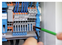
Conductor termination
