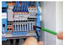
Conductor termination
