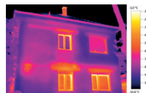
Thermal image with ScaleAssist
