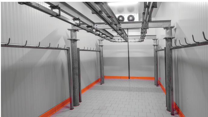
Cold Room and Storage
