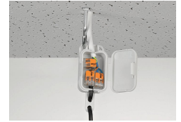
Pendant light connection in a suspended ceiling
