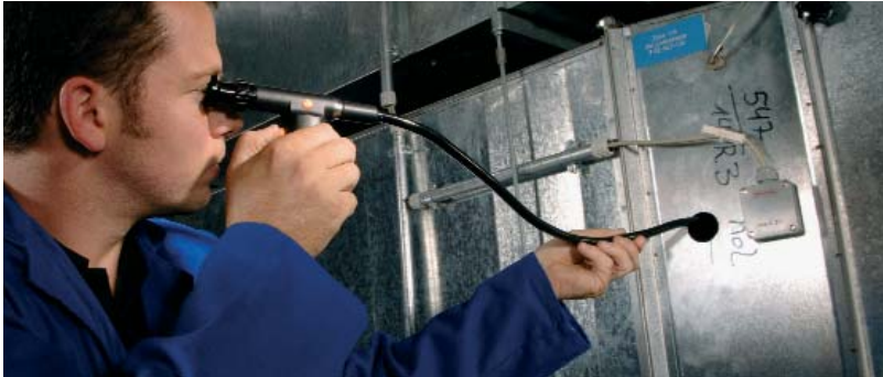
Checking in an air conditioning duct with gooseneck covering, medium flexibility.
